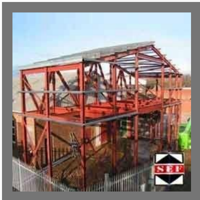
Structural Fabrication & Erection Services
