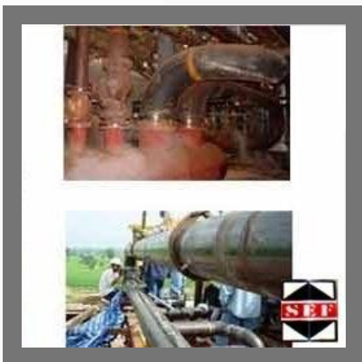
Pipelines With Fabrication & Erection Services
