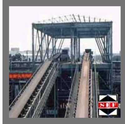
Conveyor Fabrication & Erection Services
