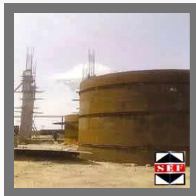
Tanks With Fabrication & Erection Services
