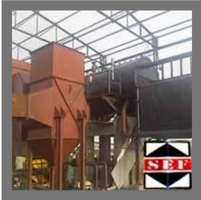
Boiler Erection & Repairing Services
